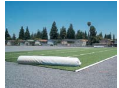
▶ Installation of synthetic turf field
