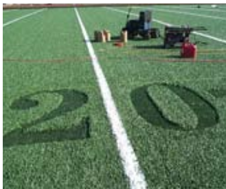
Football field: installation of yard line numbers
